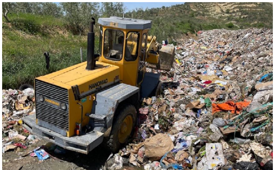
Creation of working face for appropriate operational layering and compacting waste
